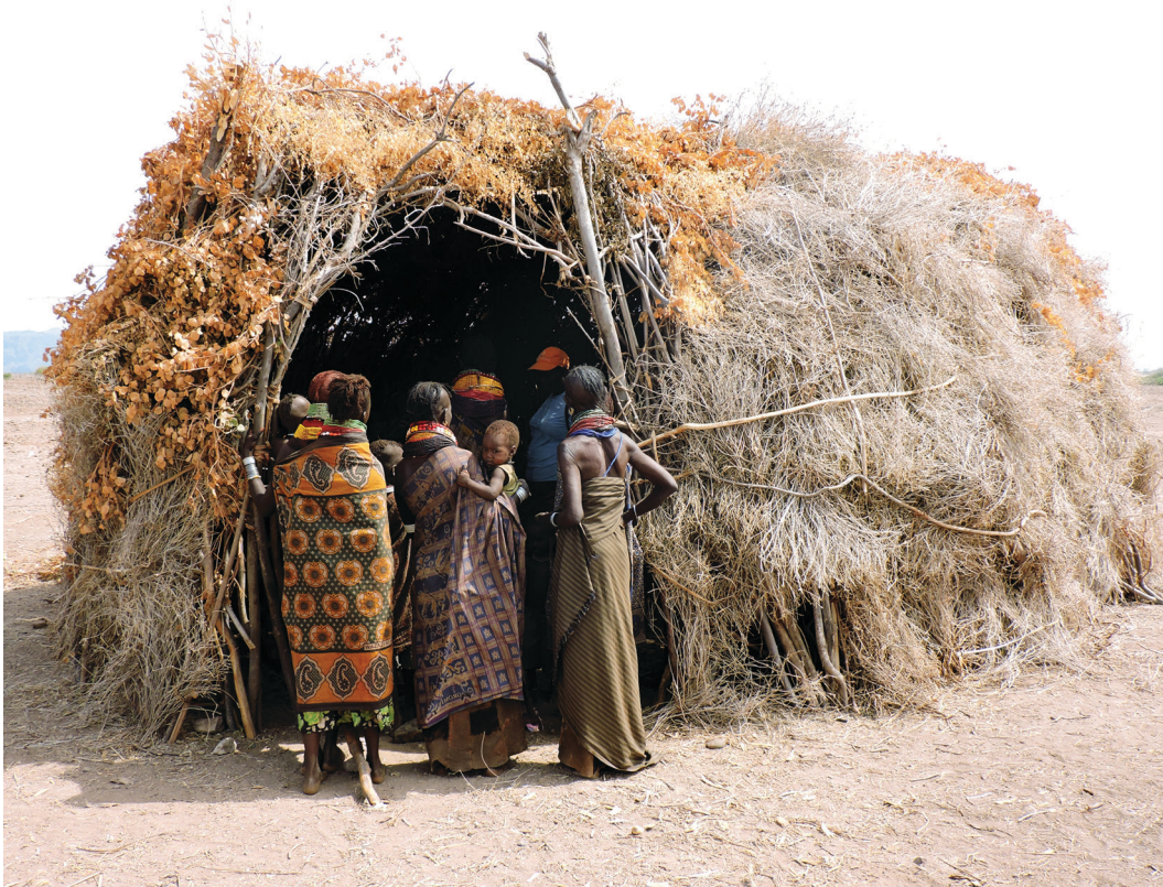
Figure 2. Communal Manyata (hut made of mud, clay and acacia or Esekon branches, created for communal use and food distribution by non-governmental organizations). Turkana tribe, Ilemi Triangle, Kenya, 2014.
